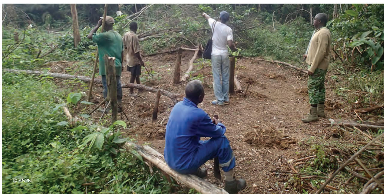
Construction site of an electric barrier
