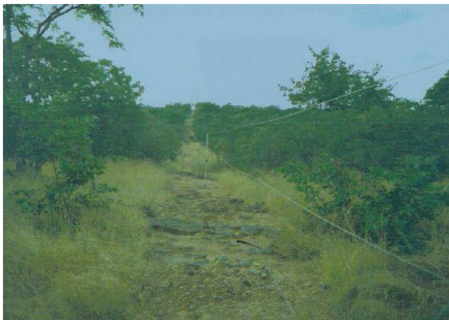
Plate 4: Example of a well-cleared line, Tyunga Ward, Binga District. Large sections of this fence are not working due to flood damage. Note low tension of fence wires caused by animal damage as a result of no electrical current.
