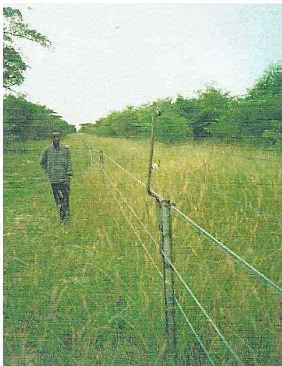
Plate 5: Example of cost-cutting measures used to modify an existing veterinary control fence, Tsholotsho Communal Land. Elephants have rendered this fence inoperable after bending the steel extensions carrying the electric wires.
