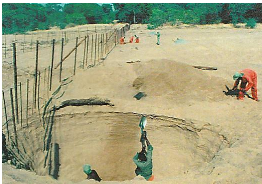
Plate 11: River crossings present problems for electric fencing. In this case, a "curtain" is being constructed to accommodate flash floods.
