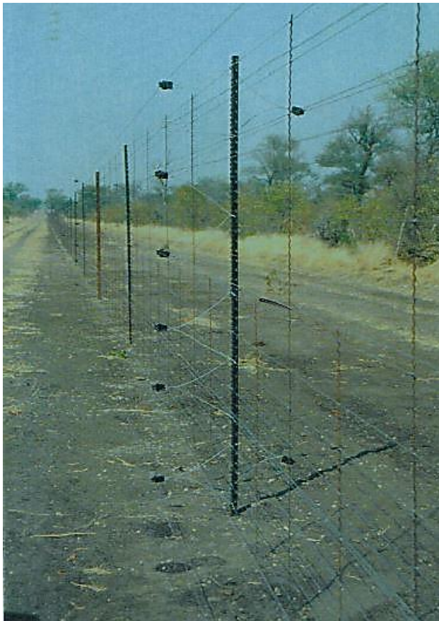
Plate 10: Two metre high electric fence carrying six live wires. Note cleared service road and lack of vegetation
